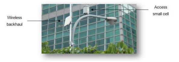
Figure 4: Sub 6 GHz Deployment on a Lamppost
